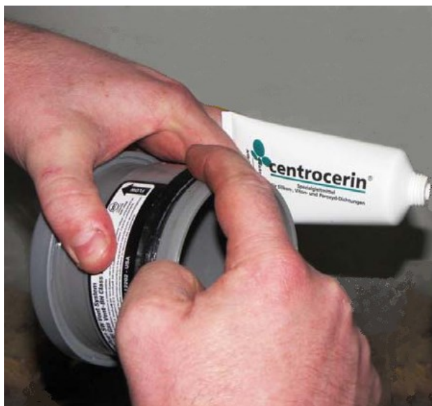
Figure 5: Applying Lubricant to Gasket
